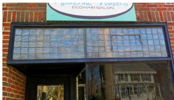
Early 20th century prismatic glass admits light above an entry door.
