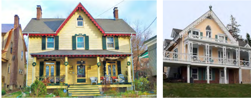
Forms and details such as rectangular massing with a cross-gable and simplified vergeboards identify Folk Victorian homes.
