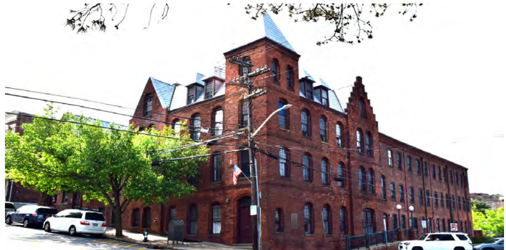
Burnham Building on South Astor Street
