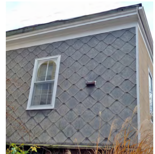
Some unusual vintage materials remain in the District, like the diamond patterned asphalt siding above. Though perhaps not original, they might be retained where restoration of the original wood siding is not possible.
