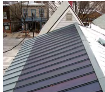
Low profile integrated solar collector
