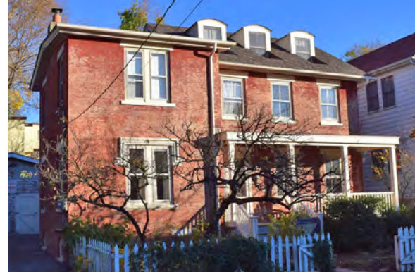
A brick masonry Italianate example with a low-pitched roof, and tall, narrow paired windows topped with a decorative crown on the first floor.
