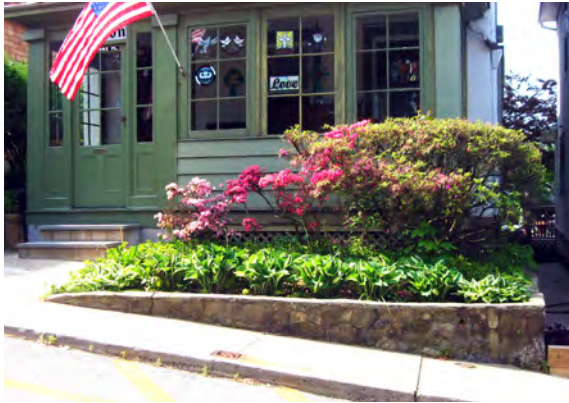
Mortared retaining wall.
