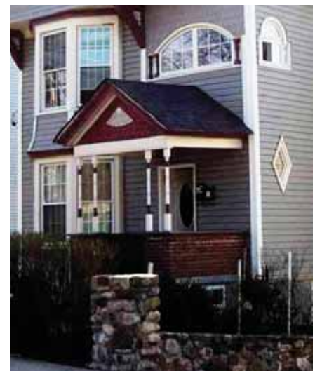
An otherwise successful portico entry is marred by the inappropriate use of masonry cheek walls where there should be a railing.
