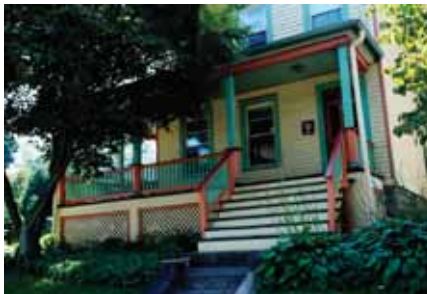
Low plantings in the 19th c. manner reveal house & porch details.
