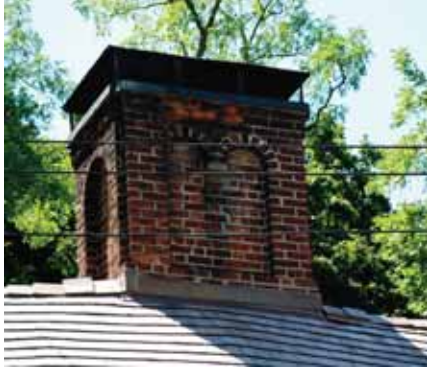
The retention of the arched insets and base flashing are good. The metal cap should be smaller.
