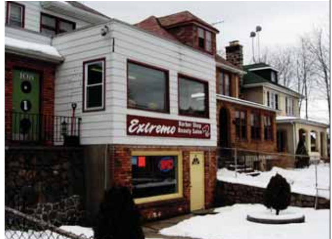
This commercial addition does harm to the context.
