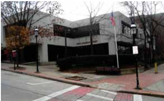
LEFT: The L-shape of this mid - 20th century building bears little relation to the aligned front-ages across the street. A dense hedge prevents the open space created from relating to the Aqueduct Trail it overlooks to the right.
