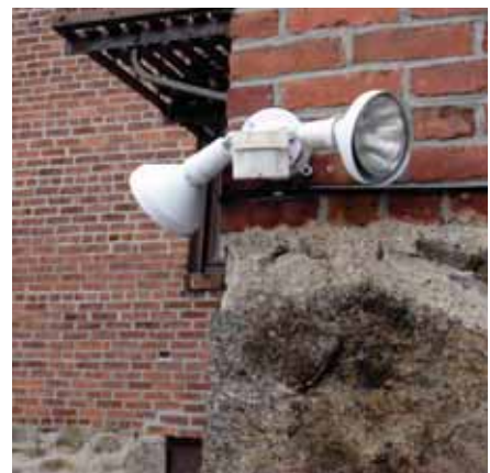
Spotlight should be deeply shielded and mounted high to prevent glare that can endanger motorists.
