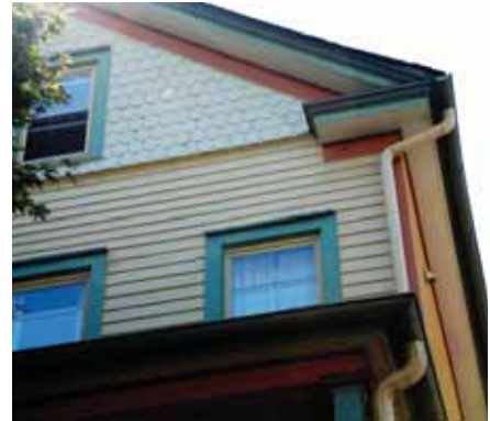
Well tended historic shingling and a carefully executed color scheme work together-note gutters and leaders painted to match siding & trim.
