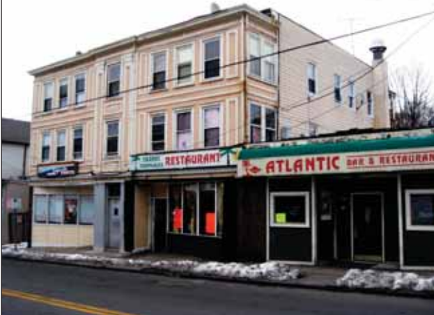
Scale shifts are abrupt along Croton Avenue; continuity at street level should be promoted.
