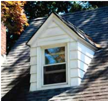
This traditional gable dormer has a good scale; the valley and sidewall flashings should be improved.
