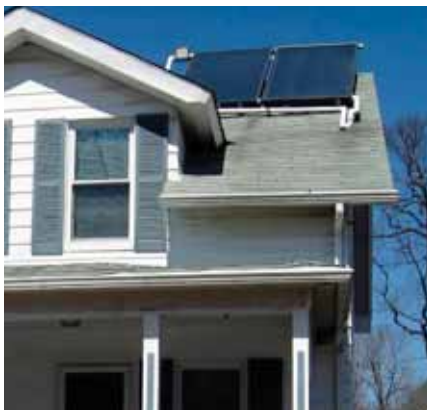
Equipment placement could be better integrated with the building.
