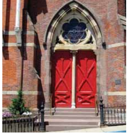
Successful historic entries consist of an assembly of elements including railing, step, molded surround and finally the doors themselves.
