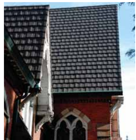
The coated metal substitute on the First Baptist Church roof differs from the original slate but has texture, shadow and a long life.
