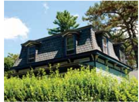
The original pattern & scale of roof materials enhanced the roof forms. Substitute materials like the “shadow” shingles above should be judged case by case. Studies show that original materials like slate and copper are the LEAST expensive on a life cycle basis.
