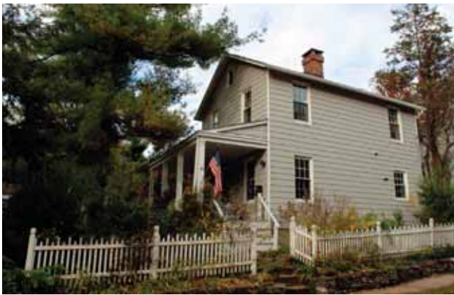
Regular repainting or restaining will protect this appropriate picket fence.
