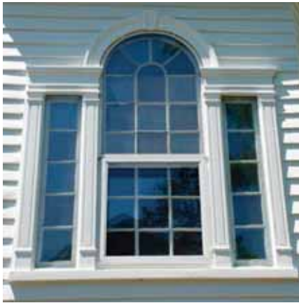
There are many historic round-top windows, but they have been over-used in renovations.
