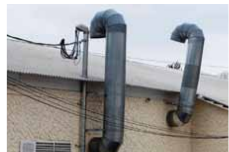
Mechanical systems should be concealed to the extent possible
