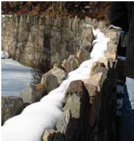
This 20th c. masonry wall was a favorite in the Hudson valley suburbs.
