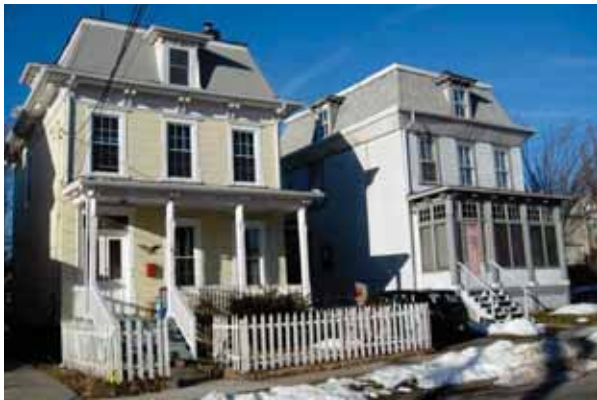
Sisters under the Skin: The building on the right probably has the original eaves bracket detailing hidden--and well preserved--under the blank aluminum soffit.
