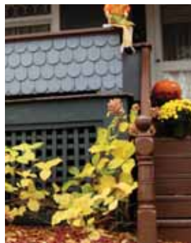
Lattice is best employed on buildings in a framed panel as at left, not as architectural wallpaper as at right.
