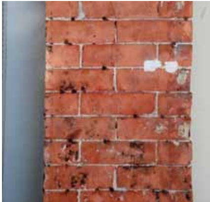
Historic masonry needs special care. See masonry section & appendices
