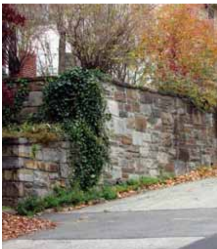
Weep holes at base of large retaining wall relieve water pressure.
