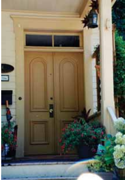
Original detailing can survive with good maintenance.
