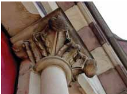
Wasp nests & biological growth compound the damaging scars of amateur repairs, wasp nests, and weather.
