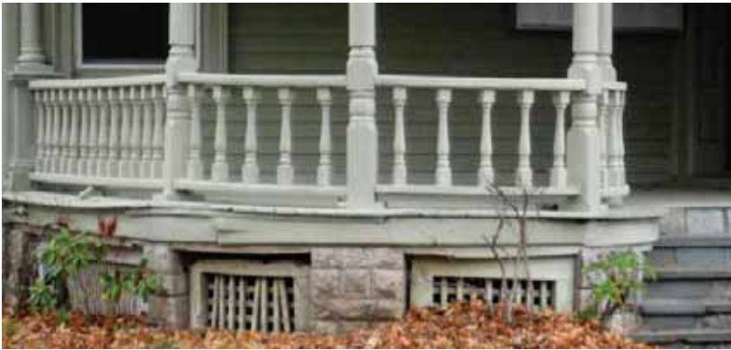
A careful search of older Village structures and documentary sources is rewarded with examples (above) of original lattice patterns: organized on a horizontal and vertical grid, densely spaced and in framed panels.
