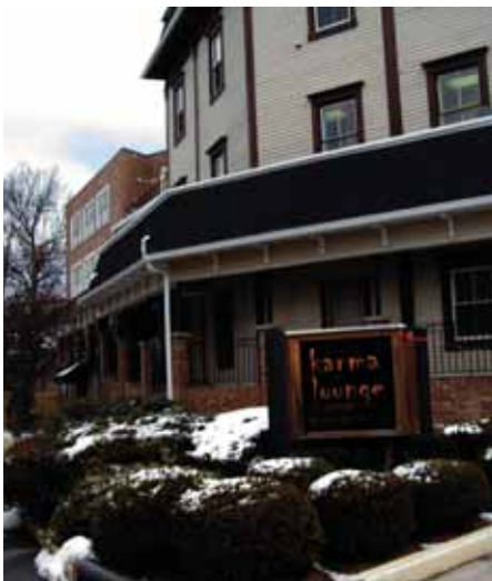
LEFT: Anachronistic and insensitive details such as brick piers, wrought iron railings, and white gutters and leaders compound the problems created by trying to fit a massive new element such as this covered walkway into an historic context.
