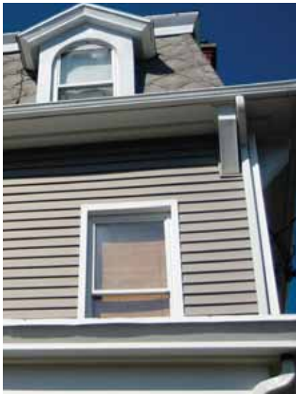
Gutters and leaders should be tidy and match siding and trim colors and conditions.
