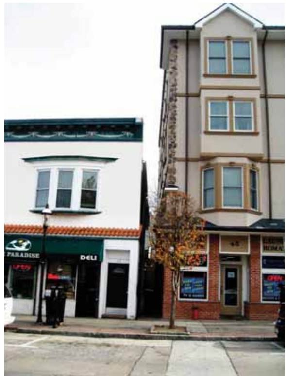
RIGHT: Introducing rustic materials like the stone quoining on the right, where they don't otherwise exist, can strike a false note.
