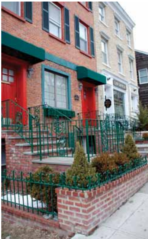
LEFT: Comfortable scale, material and a few simple details can help new build- ings relate to their context.
