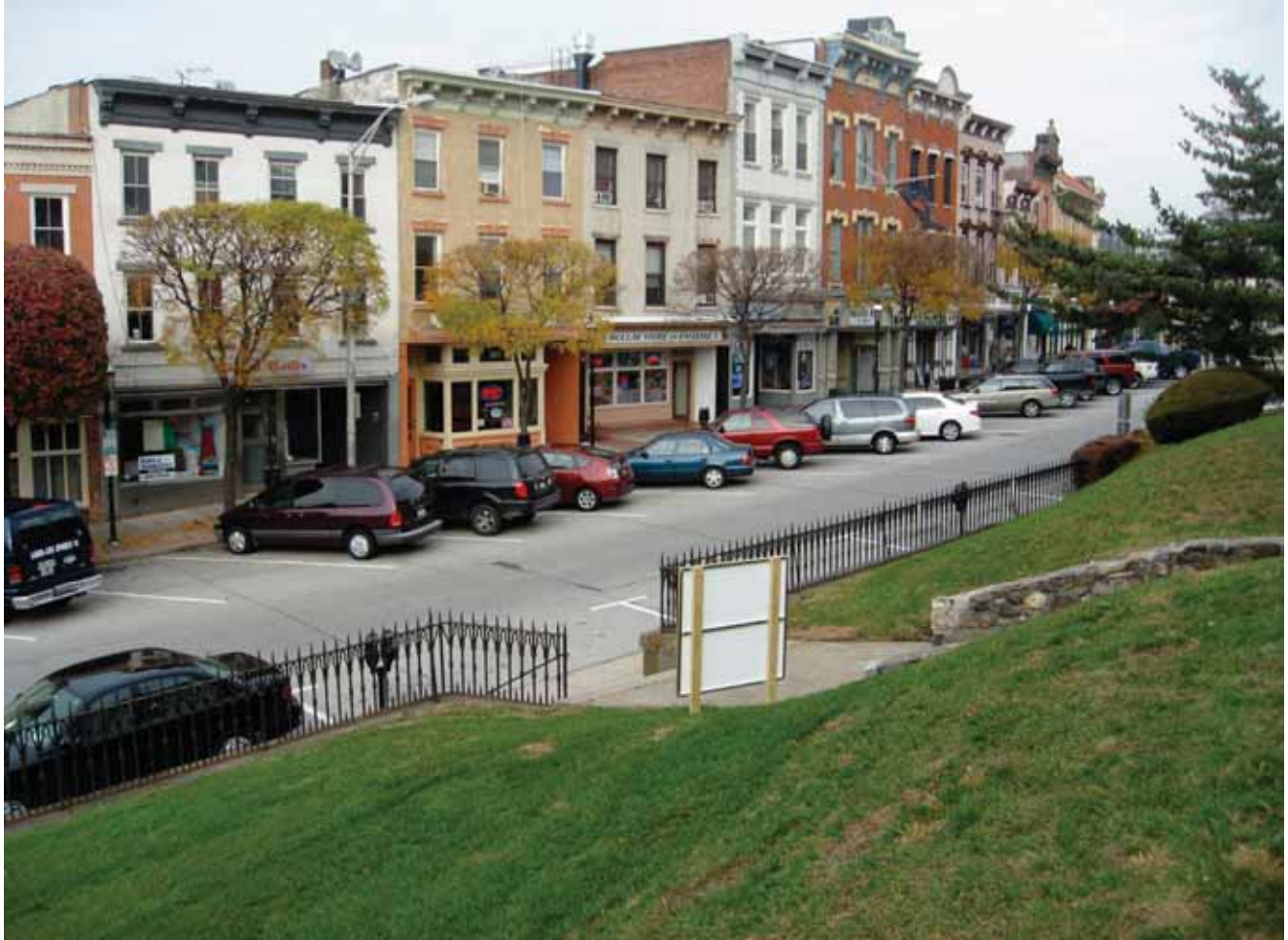
A row of vintage facades is visible from a vantage point on the property of the 1874 First Baptist Church
