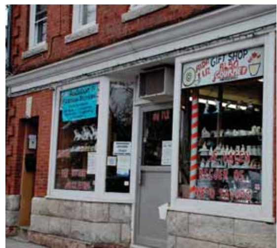
RIGHT: A recent door (and the AC unit overhead) is a jarring note in this solid historic storefront housing a variety of useful services.
