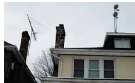
Antennae create clutter and can provide entrance points for water.
