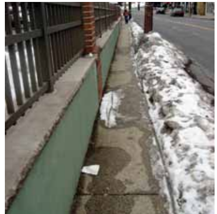
This little strip makes it hard to walk to the shopping center.
