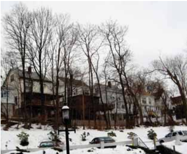
Residential porches overlook unscreened parking lot.
