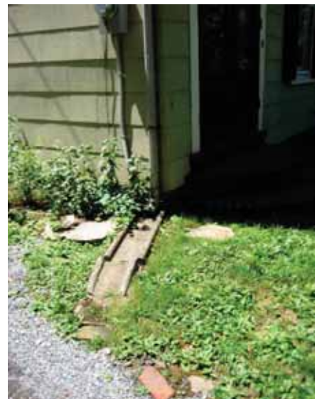
Unscreened splash block.
