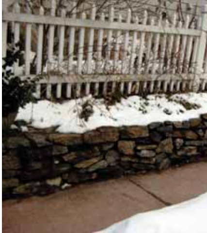
Low dry-laid wall provides excellent drainage for garden bed.
