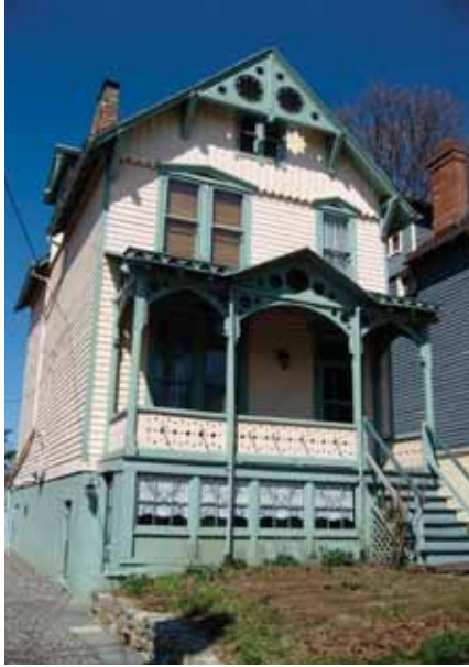
Exuberant wood detailing and surfaces require skilled repairs.
