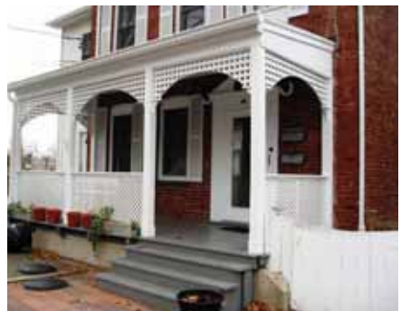
Lattice is best employed on buildings in a framed panel as at left, not as architectural wallpaper as at right.
