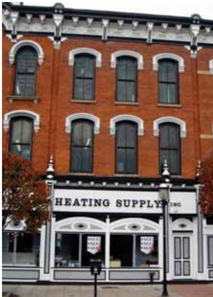
Signage can be an important part of an overall facade treatment and color scheme.
