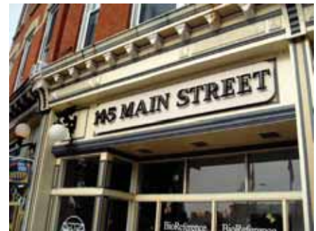
The original punched transoms strengthen the sign panel above and send daylight further into the space.
